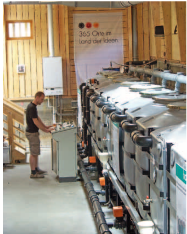
Figure 2: Greywater recycling plant in the residential complex “Block 6” in Berlin. Photo: E. Nolde/Flickr
