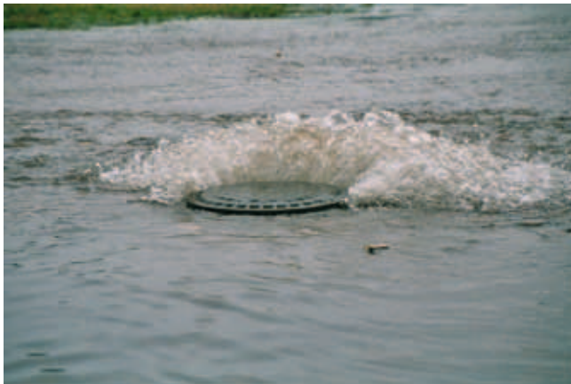
Figure 1: Heavy rain can overload sewer networks and lead to flooding. Photo: Lothar Fuchs, itwh
