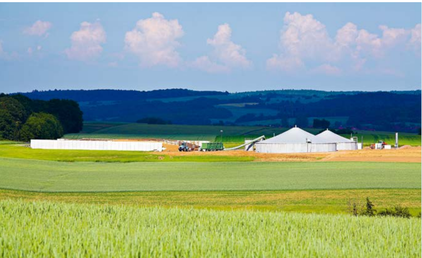
Biogasanlage in Rosenberg
