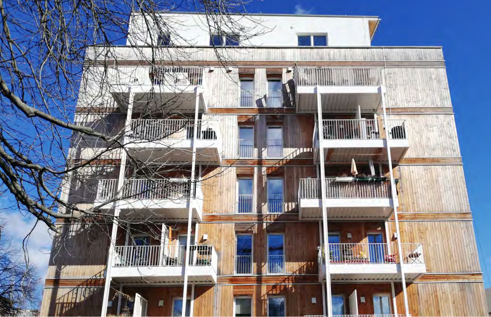
Apartment building made of timber
