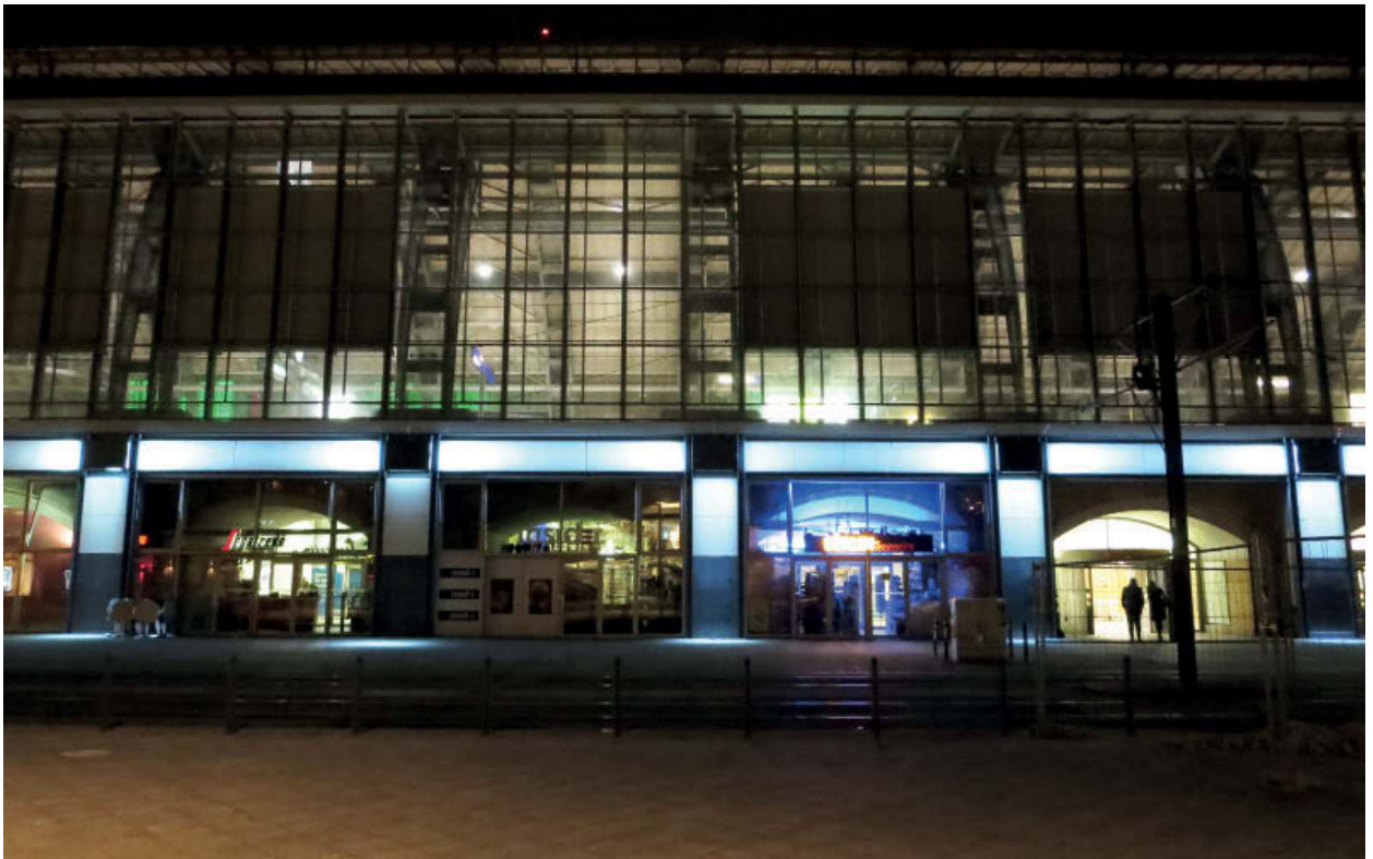
Figure 1: Bad lighting at Alexanderplatz 3 (Photo: C. Kyba)
