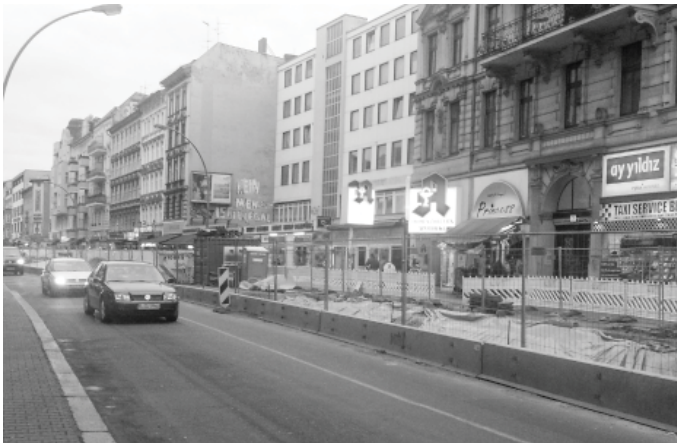
Figure 3: Urban renewal construction site (Photo: A. Steigemann 2015)
