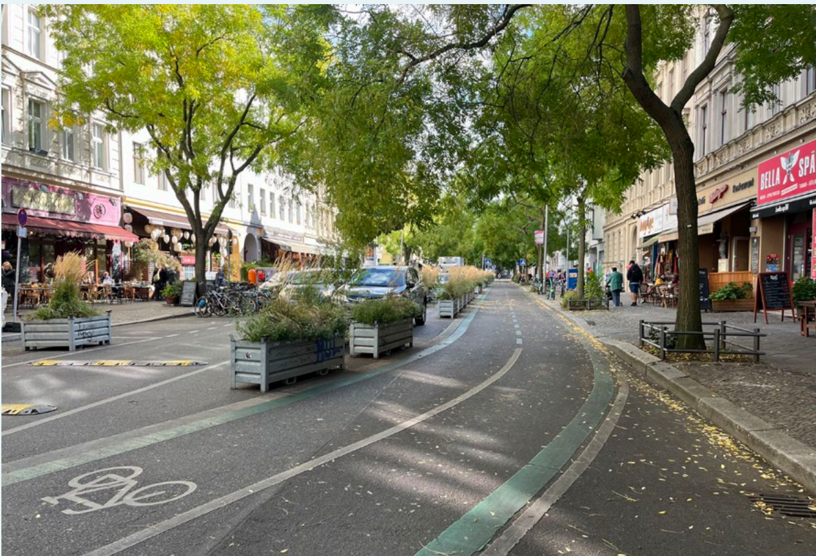
Figure 5: A two-way bicycle lane is separated from vehicular traffic with planters. Temporary speed bumps help to calm traffic.
